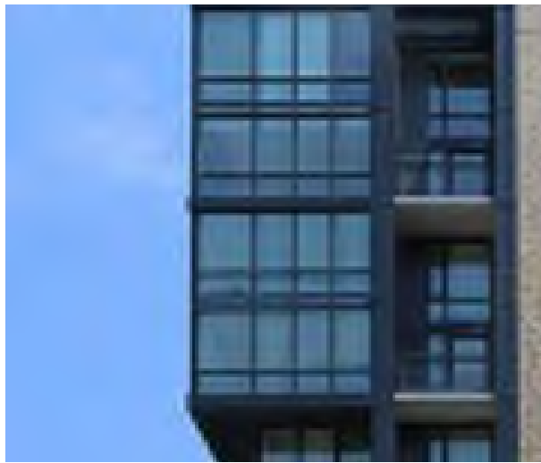
Facade A Window Wall
